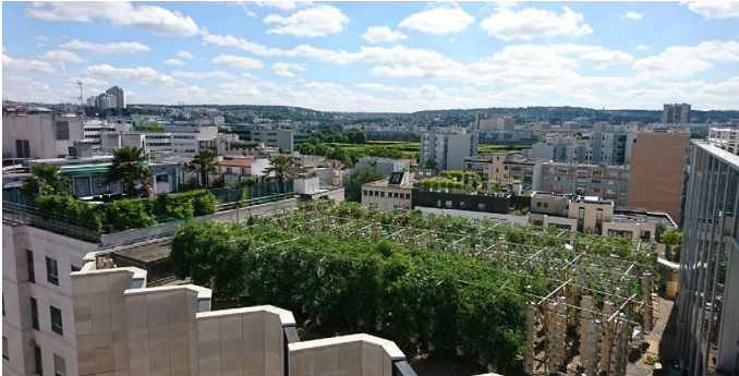
URBAN FARM IN HOTEL ROOFTOP. BOULOGNE, FRANCE
