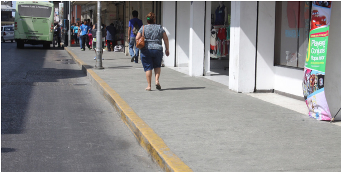
CONCRETE SIDEWALKS AND STREETS
