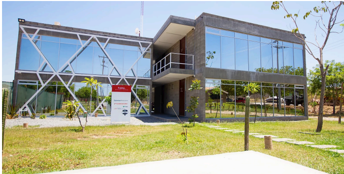
TARA OFFICE SPACE IN LA PRIMAVERA INDUSTRIAL ZONE
