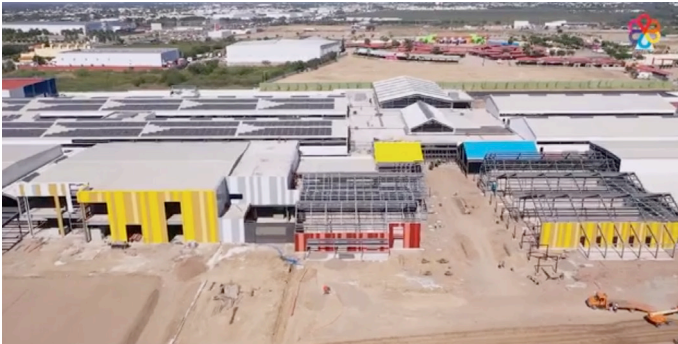
EXPLANADA SHOPPING MALL IN PROCESS
