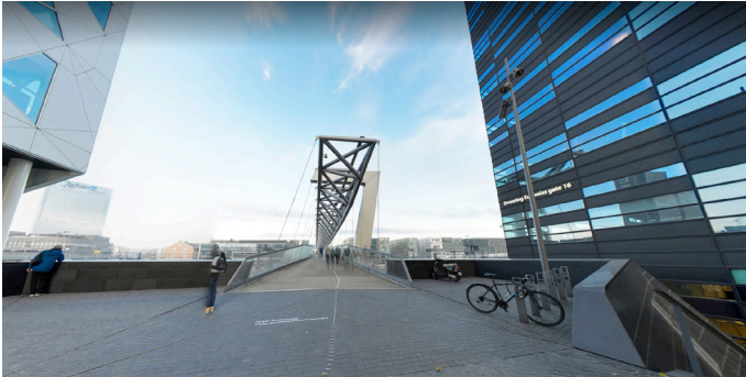
OSLO, NORWAY. PEDESTRIAN BRIDGE.
