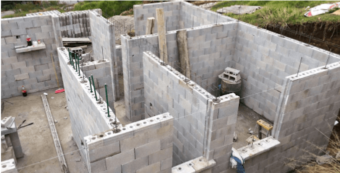
CINDER / CONCRETE BLOCKS
